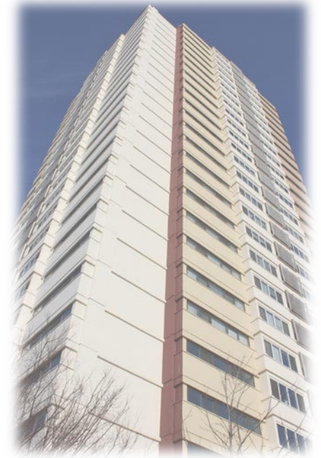
Courtyard Apartments Philadelphia, PA
